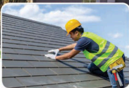
Roof Analysis & NO-LEAK Certification
