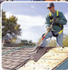
Leak & Damage Repair
