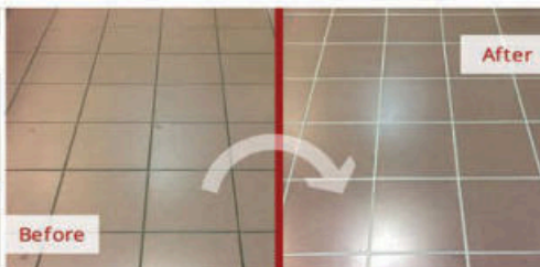
Grout & Tile Sealing
