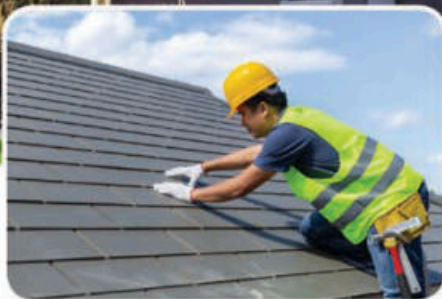
Roof Analysis & NO-LEAK Certification
