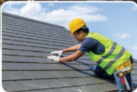
Roof Analysis & NO-LEAK Certification
