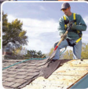
Leak & Damage Repair
