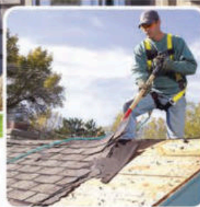
Leak & Damage Repair
