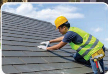
Roof Analysis & NO-LEAK Certification
