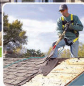
Leak & Damage Repair
