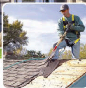
Leak & Damage Repair
