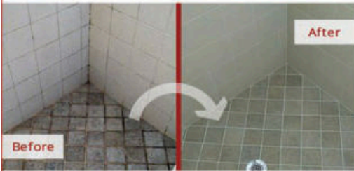
Complete Shower Restoration
