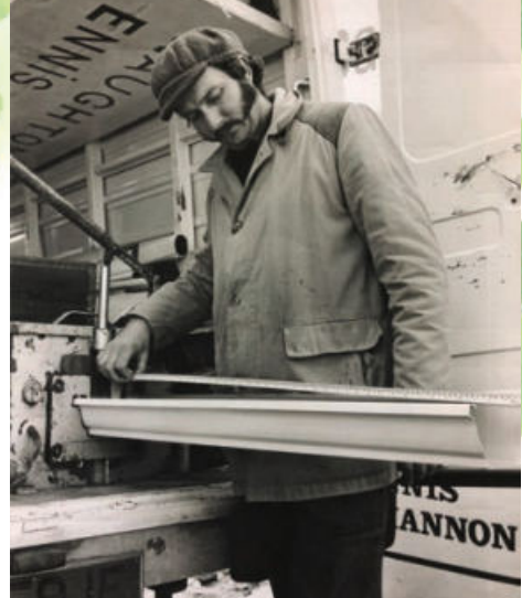
Noel's father, Patrick Naughton, installing gutters in 1976
