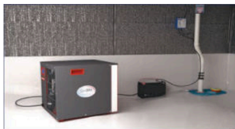
crawl space repair
