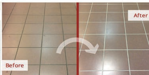
Grout & Tile Sealing
