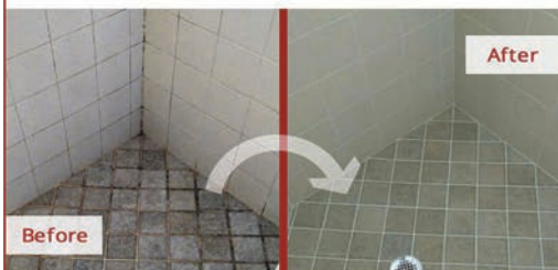
Complete Shower Restoration
