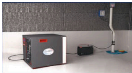
crawl space repair
