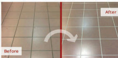
Grout & Tile Sealing
