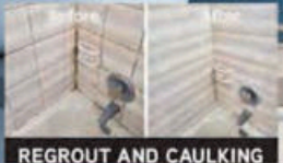
REGROUT AND CAULKING
