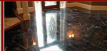
TILE & GROUT RESTORATION
